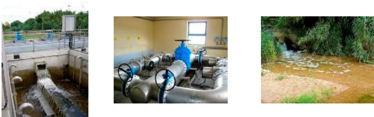
Figures 1 - 3. Pictures of the water reclamation process at Blanes and the reclaimed water produced: on the left, details of the filters; in the centre, disinfection equipment with ultraviolet light; and, on the right, picture of the point where the reclaimed water comes out in the bank of the Tordera.
